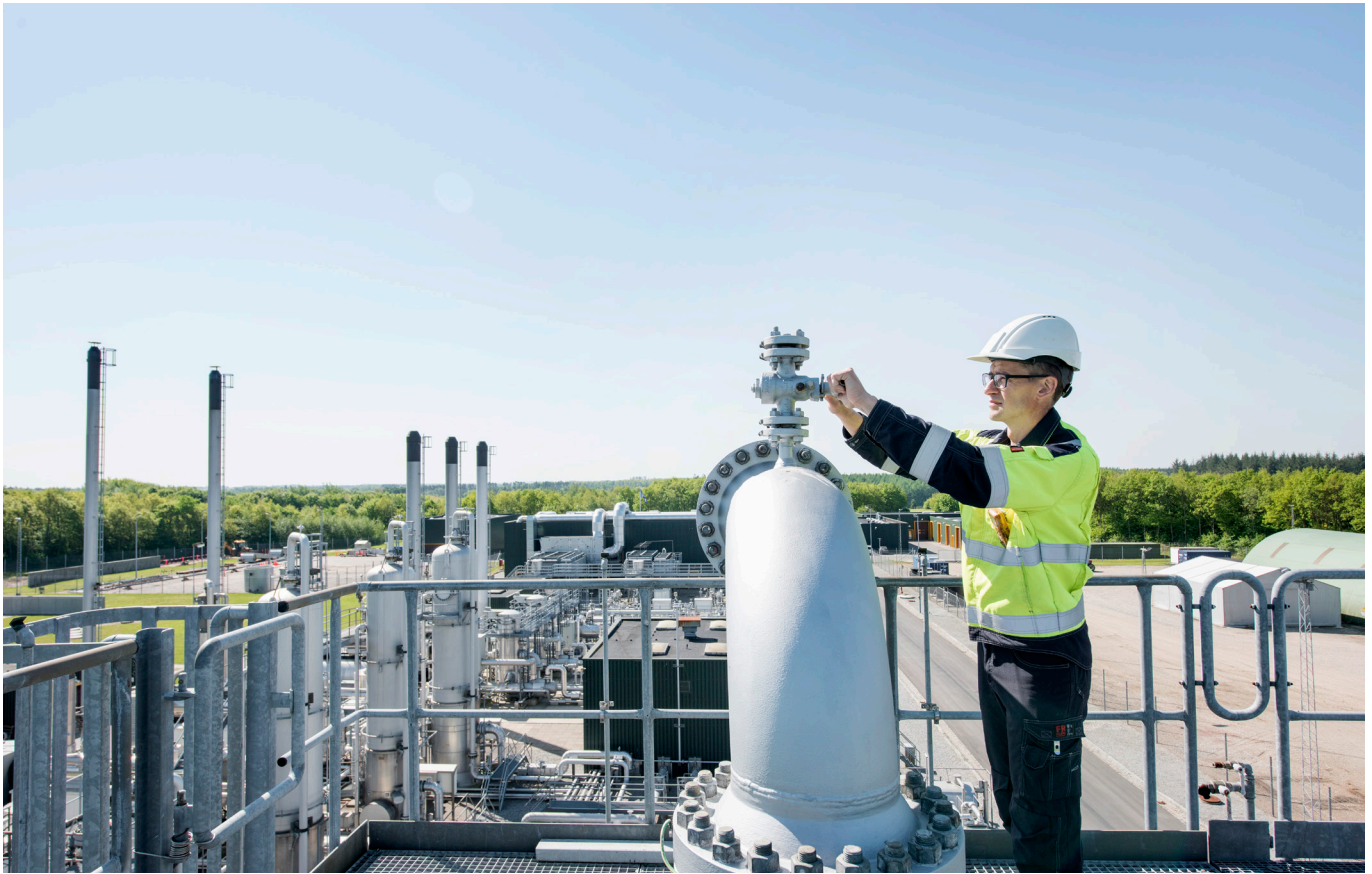
Lille Torup Gas Storage Facility
