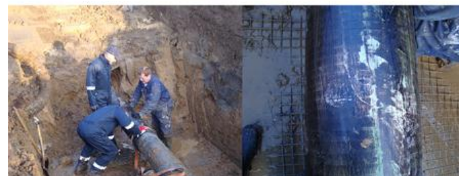
Repair work on a pipeline following pigging.
