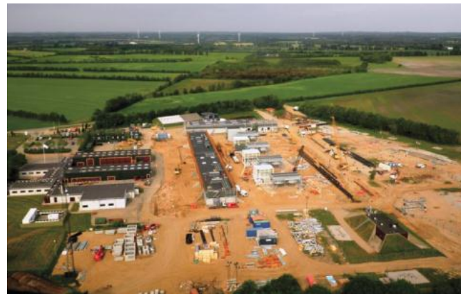
Compressor site in Egtved
