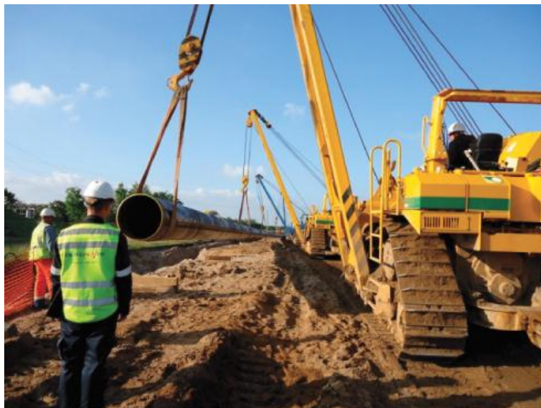
Laying the new gas pipeline.
