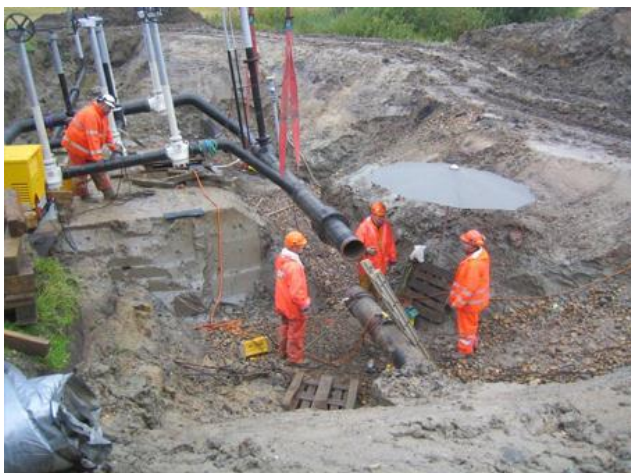
Welding in a new valve station at Sejling Hedevej.
