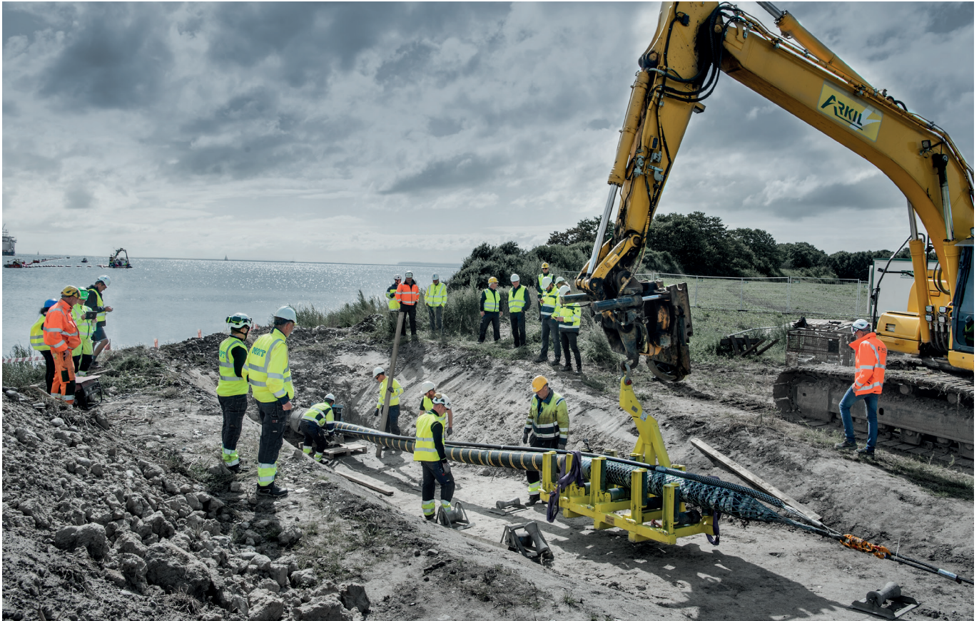
Here, the submarine cable for the EU-subsidised Kriegers Flak project is landed. The project will connect German offshore wind farms to a future Danish offshore wind farm in the Baltic Sea.
