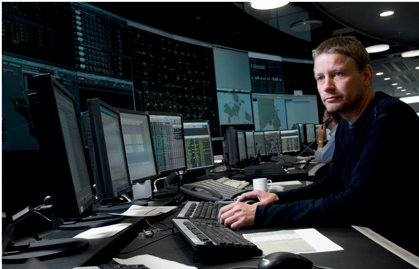
Energinet's electricity system control centre in Erritsø.
