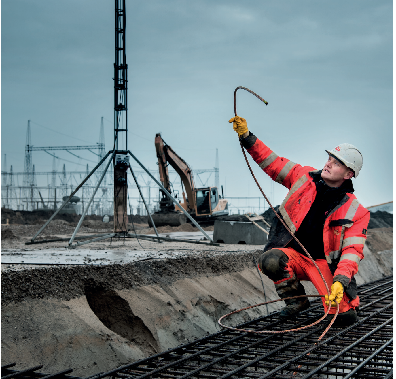
Construction of COBRACable at Endrup station in Western Jutland.
