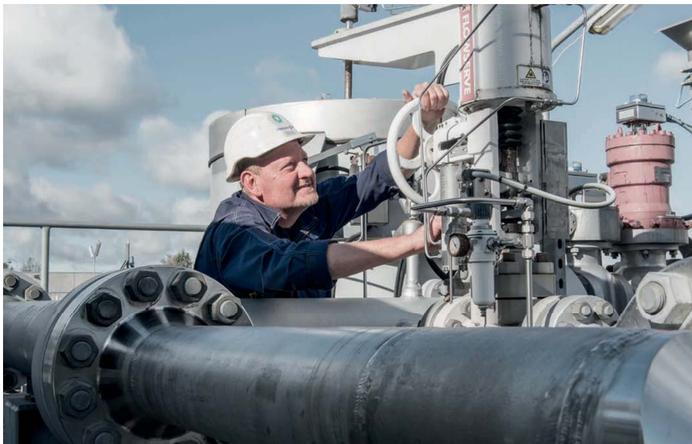
Stenlille Gas Storage Facility
