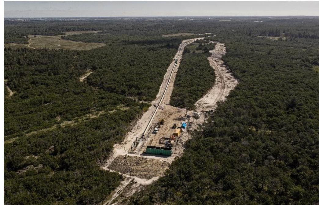
...where a pipeline of 750 meters is pulled underneath the sand dunes
