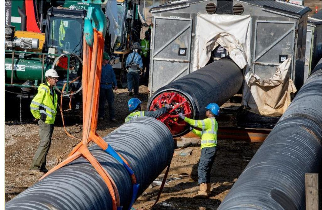
The pipelines are welded together on the Jutland side, and are then pulled across Lillebelt from the Funen side
