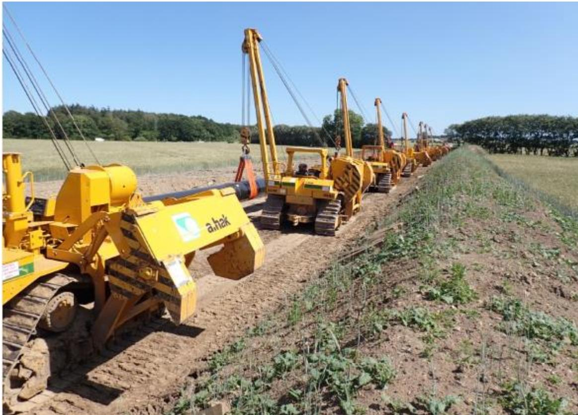
Sidebooms lifting the pipeline in place.
