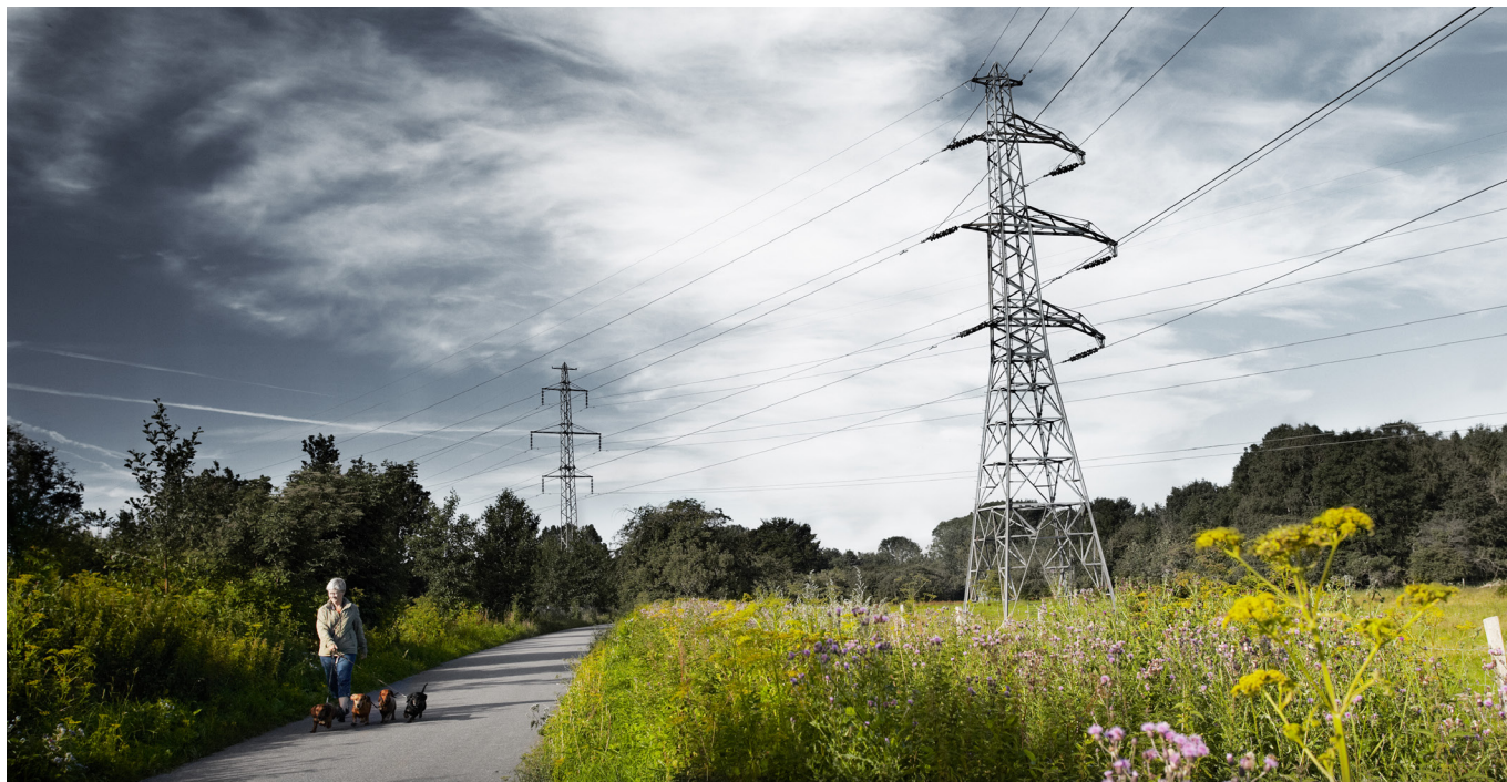
132 kV power pylons near Copenhagen.
