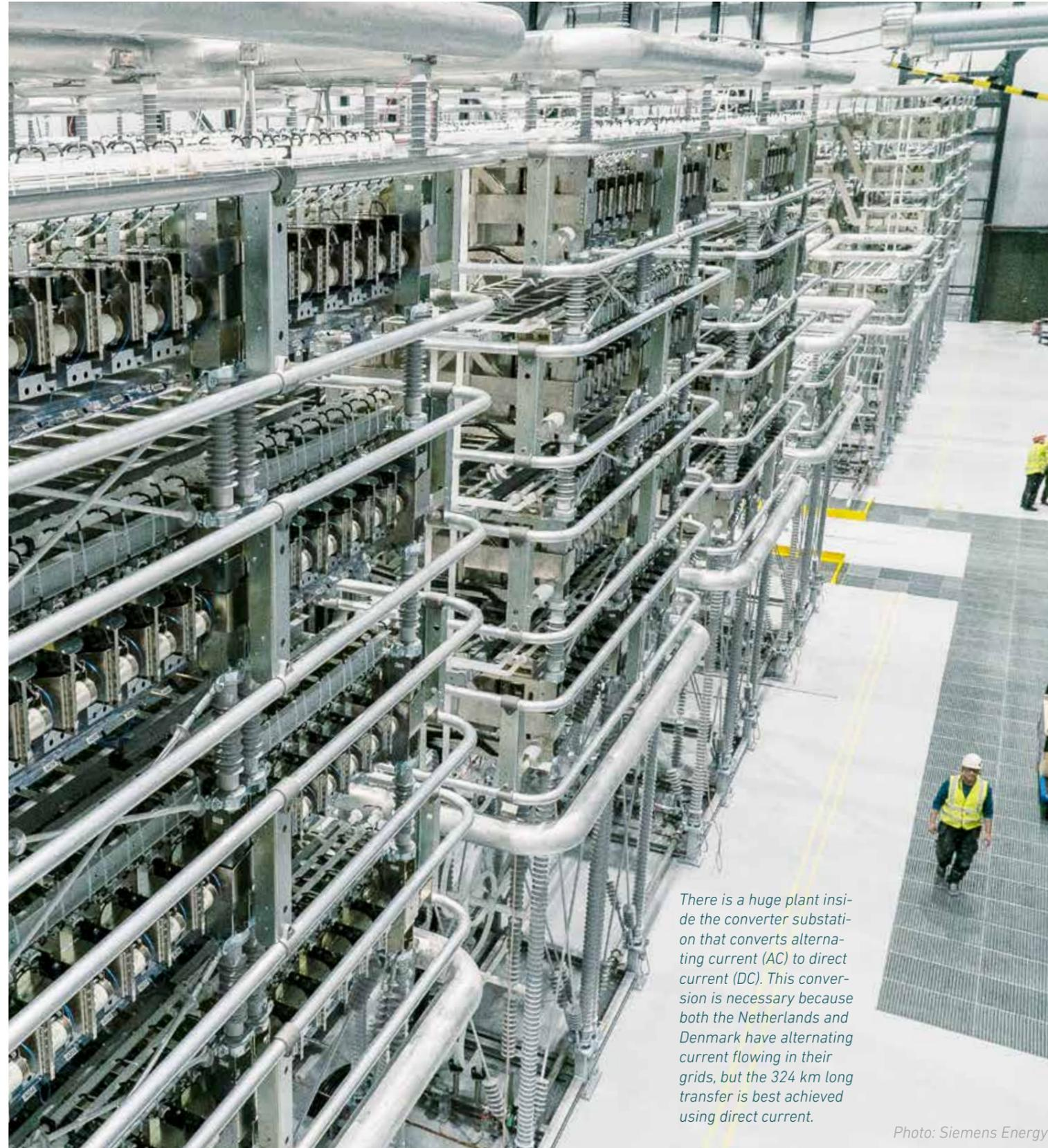
*There is a huge plant inside the converter substation that converts alternating current (AC) to direct current (DC). This conversion is necessary because both the Netherlands and Denmark have alternating current flowing in their grids, but the 324 km long transfer is best achieved using direct current.*
