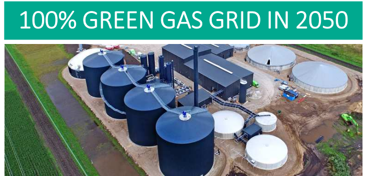
Photograph: NGF nature energy, Holsted biogas plant
