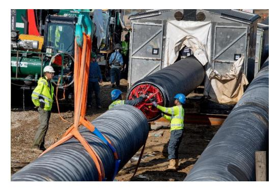
The pipelines are welded together on the Jutland side, and are then pulled across Lillebelt from the Funen side
