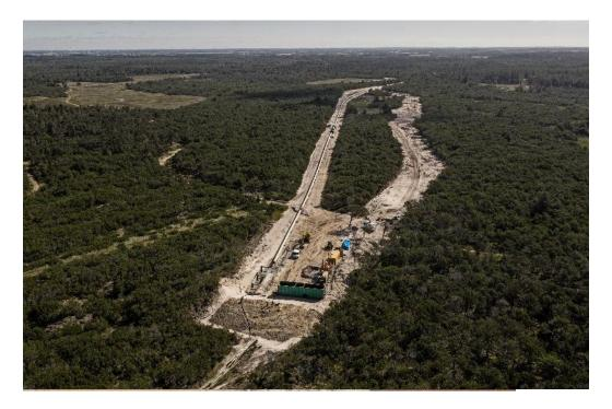
...where a pipeline of 750 meters is pulled underneath the sand dunes
